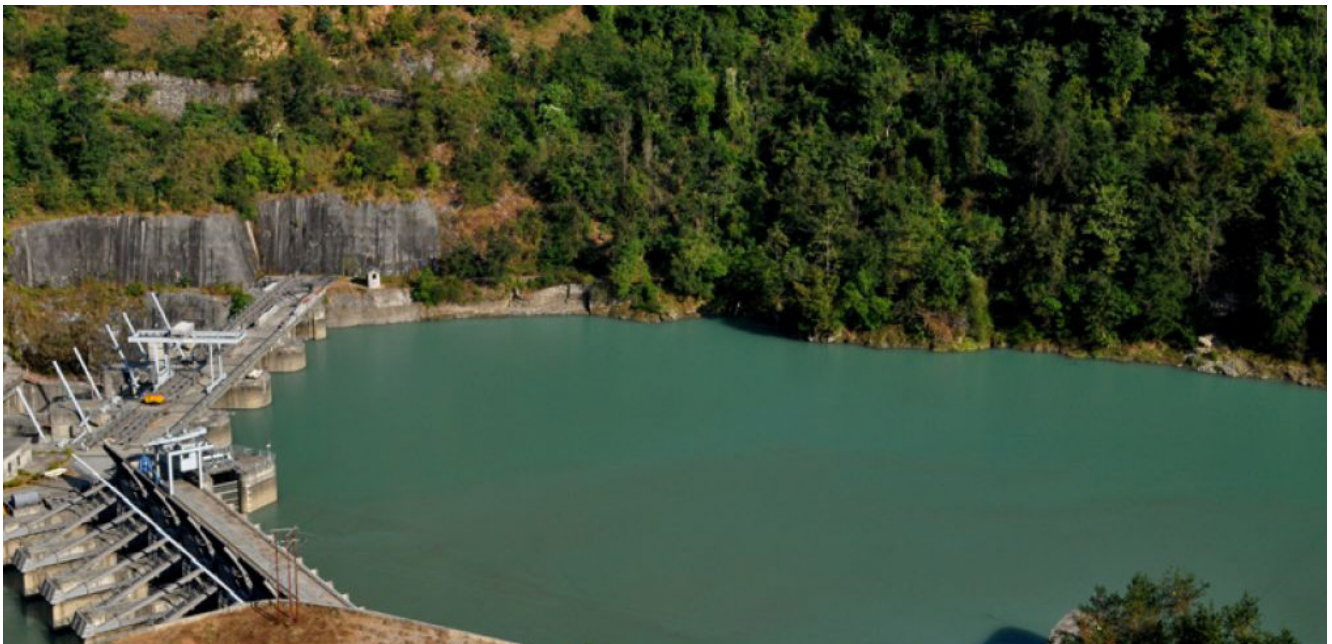
Figure 1: Kaligandaki 'A' Hydroelectric Project
