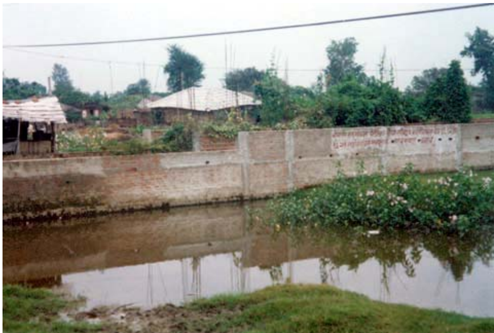
Water Logged Area
