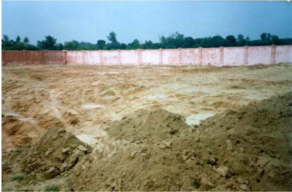
Reclamation of an Old Dumping Site
