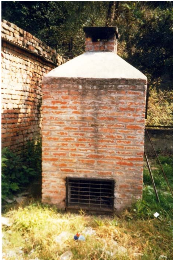
Incinerator at Bhaktapur Hospital
