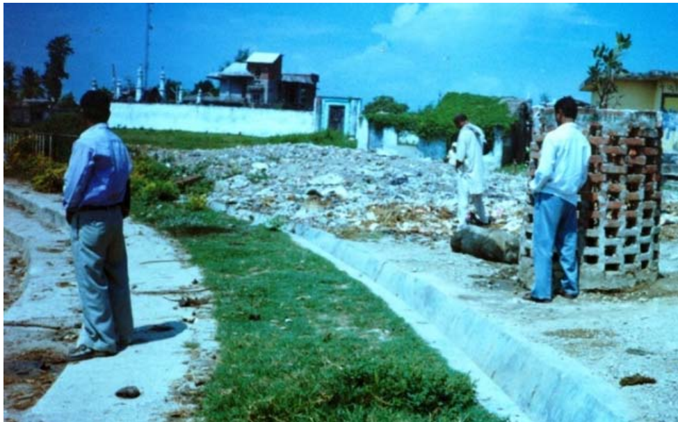
Waste Pile and Open Toilet Near a Mosque
