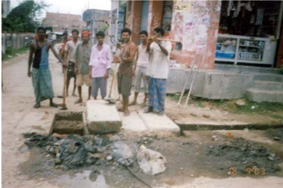
Cleaning of Drains Clogged by Waste
