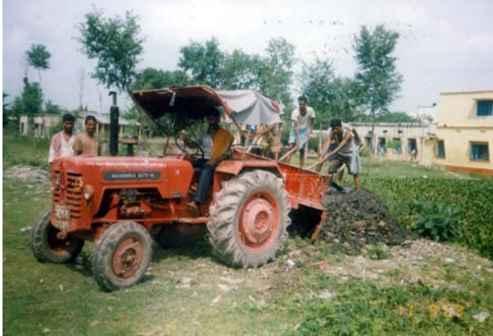
Unloading of Waste from Drains on to Open Land
