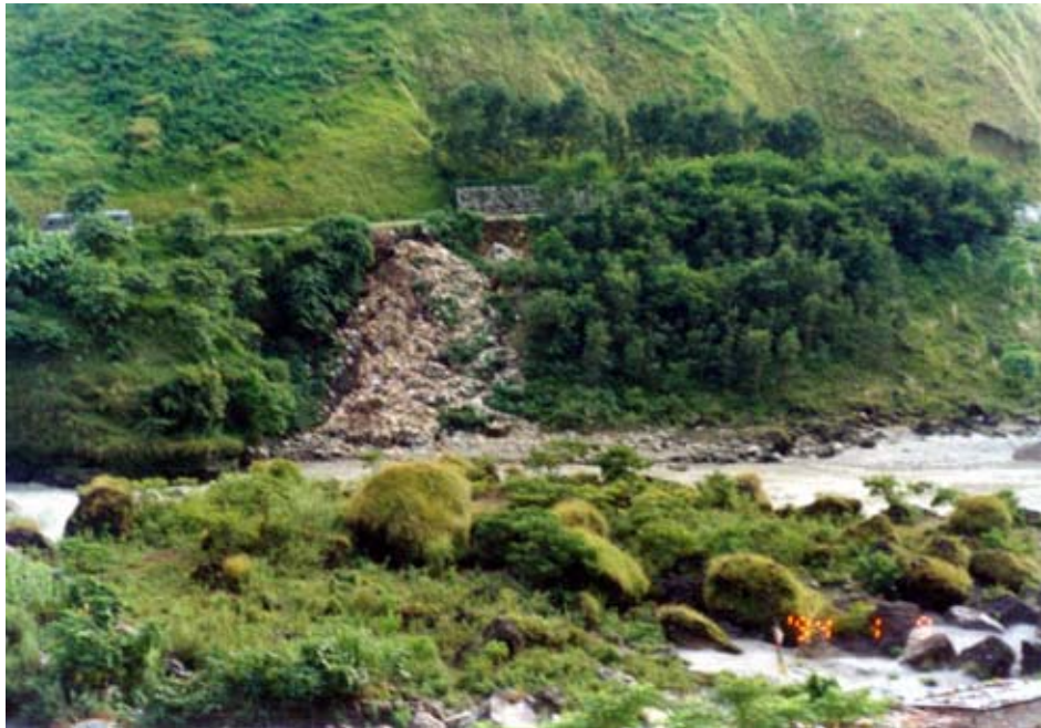
Waste Dumping Along the Highway on the Banks of Kali Gandaki River
